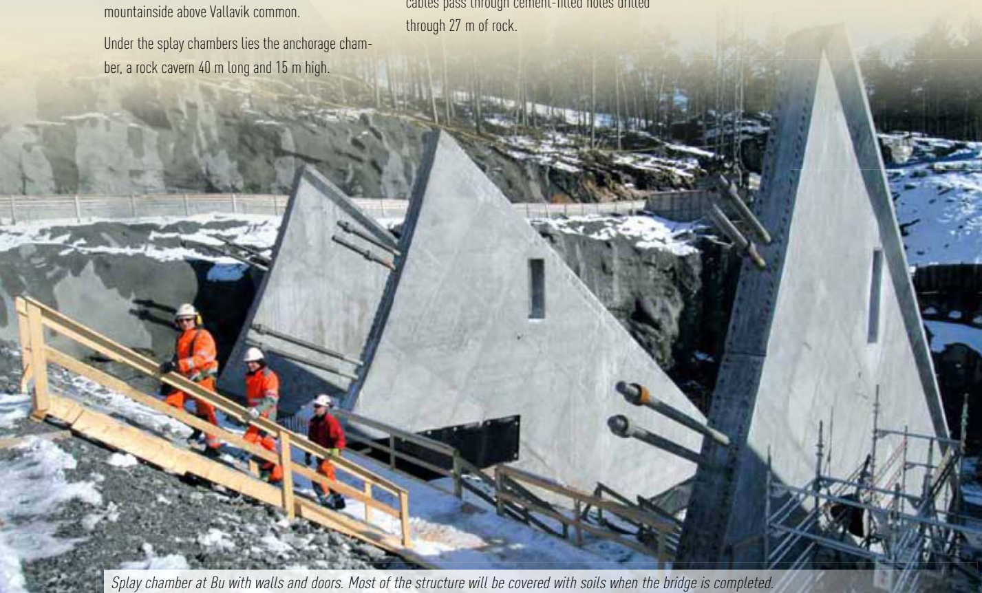
Anchorage chamber at Bu. These rock caverns are 40 m long and 15 m high.
