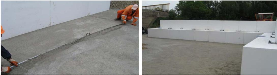
*Figure 9. Embankment grading with screed boards, prior to the setting of styrene blocks on the left, and mode of lining-up of styrene blocks on the right side*
