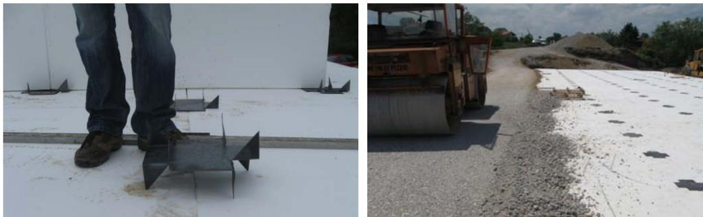
*Figure 10. Metal plate made in the workshop, which merged blocks of styrofoam, on the left and compaction of the first layer above styrofoam roller 8t, at the right*
