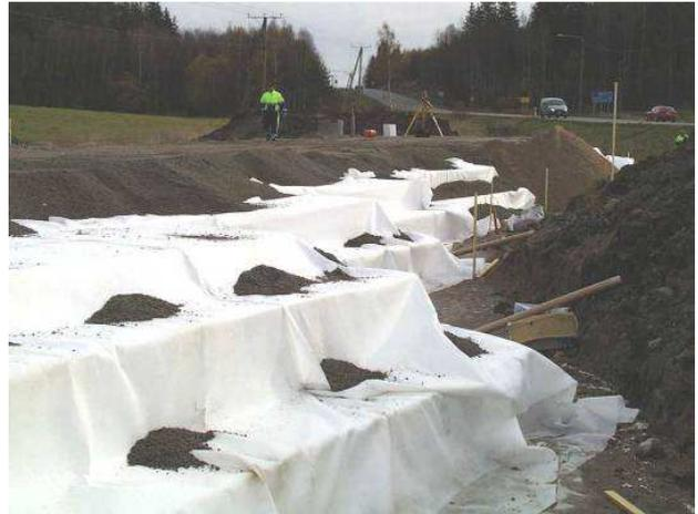
Figure 4. The covering of EPS blocks [2].
