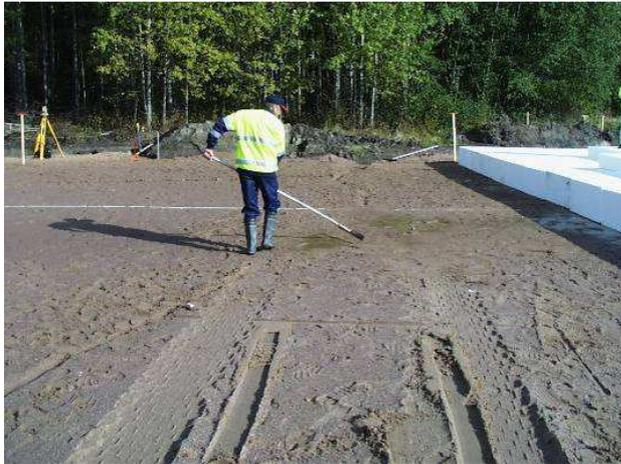
Figure 3. The preparation of levelling sand [2].
