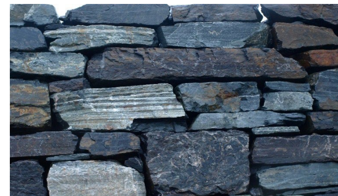
Figur 12. Prinsipp for natursteinsmur (stablemur).
