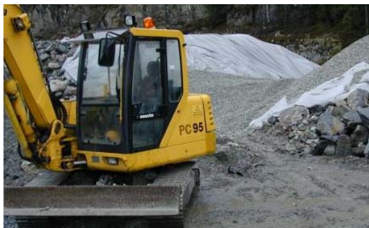
Figure 11- Light compaction of fill on diversion road at Klemetsrud
