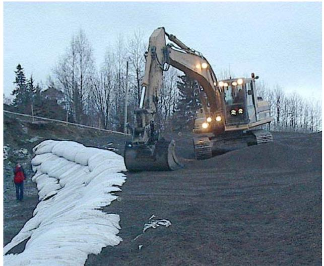
Figure 6 Digger laying LWA on the turned-up reinforcement
