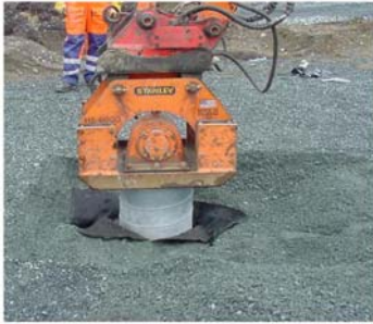
Figure 3. – Installing steel tube
