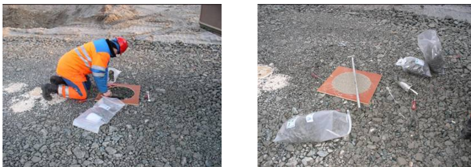
Figure 7: In place detection of density/unit weight (sand replacement method)
