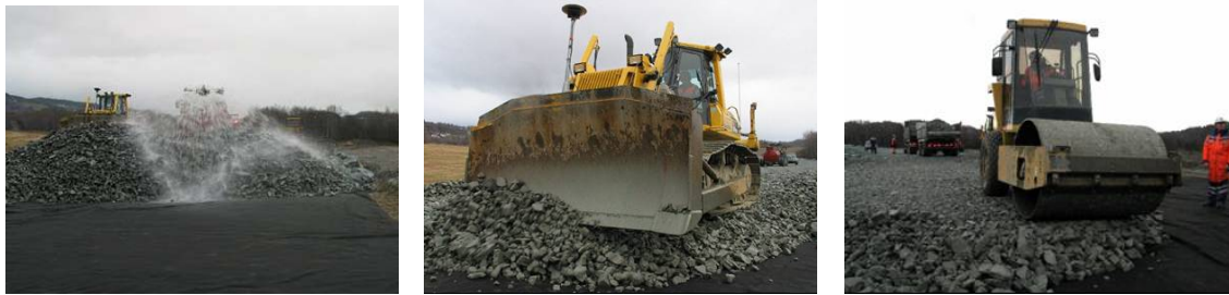
Figure 6: Sprinkling of crushed concrete materials is recommended before paving and compaction
