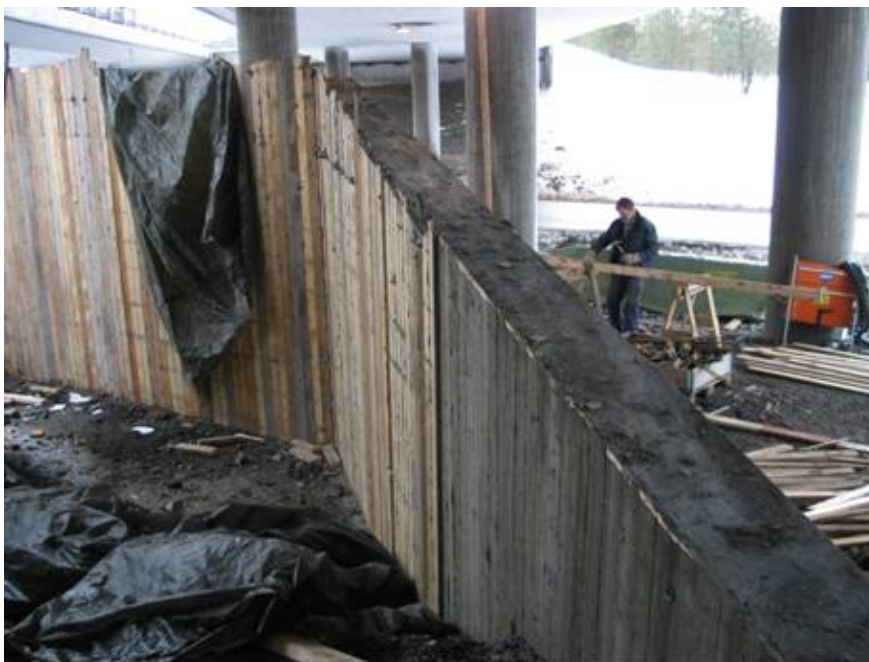
Figure 9. Retaining wall with 100% RCA in the coarse aggregate
