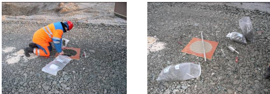
Figure 5. In place detection of density/unit weight (sand replacement method)
