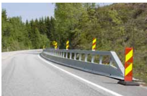
Figure 4.13 Longitudinal protection devices (examples).
