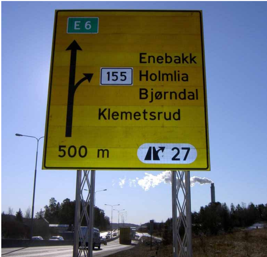
Figure 1.11 Example of an undesirable difference in colour nuance.
