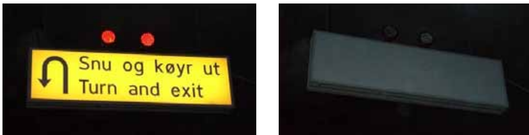
Figure 2.10 Two-position sign in active and passive positions.
