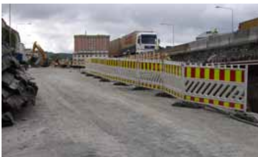
Figure 4.14 Protection devices for pedestrians and bicycle traffic.
