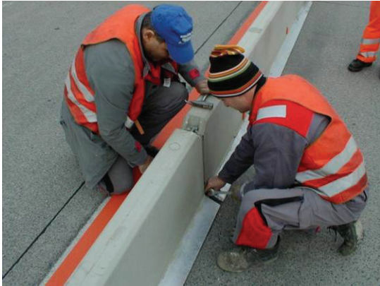
Aligning of the element and tightening the clamping bolts
