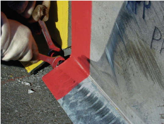
Detail: tightening the clamping bolts at the base
