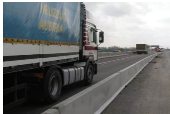
Safeguarding a construction site with containment level H1
