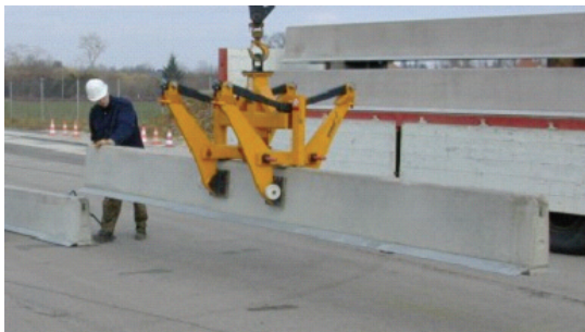
Installation with a concrete safety barrier grab
