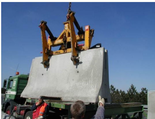
Installation using a concrete barrier grab
