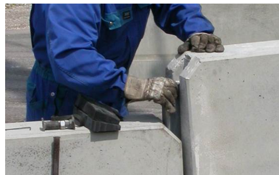
Rapid linking of the elements, using the patented coupling system
