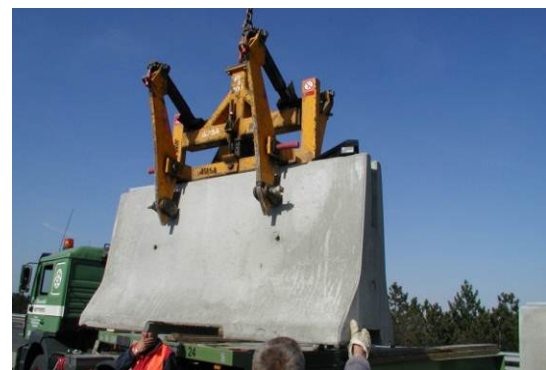
Moving the elements using a concrete barrier grab
