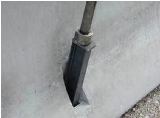
Detailed view of hydraulic hammer and steel spike
