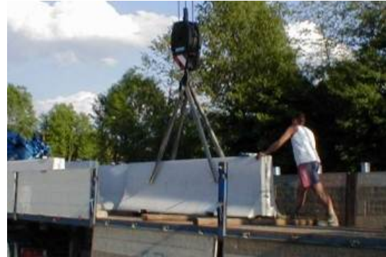
Moving the elements using straps
