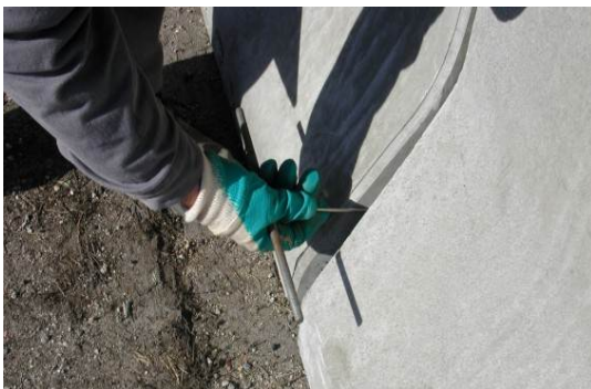
Installation of butt joint inserts
