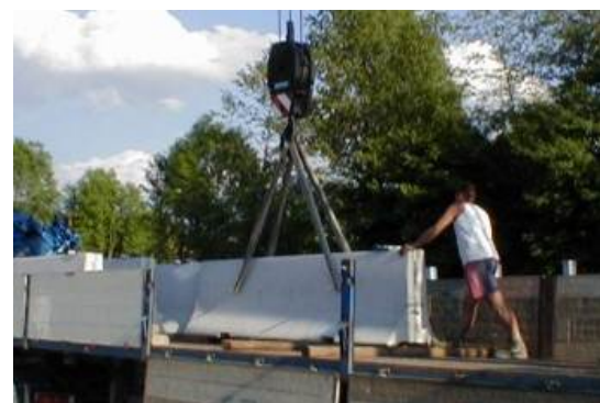
Moving the elements using straps
