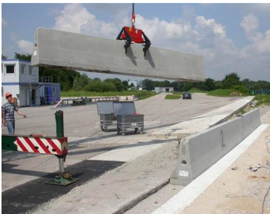
Moving the elements using a concrete barrier grab
