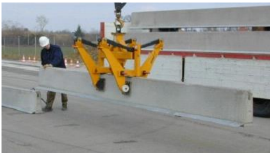
Installation with a concrete safety barrier grab
