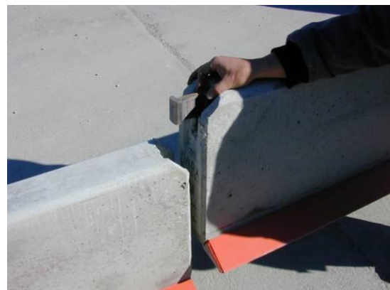
Lowering the element and inserting of the patented coupling
