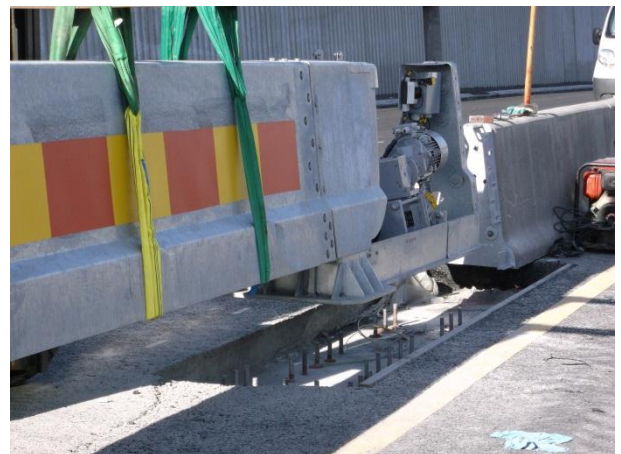
Installing CADO beam with pivot
