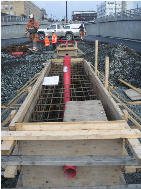
Concrete preparing CADO foundation
