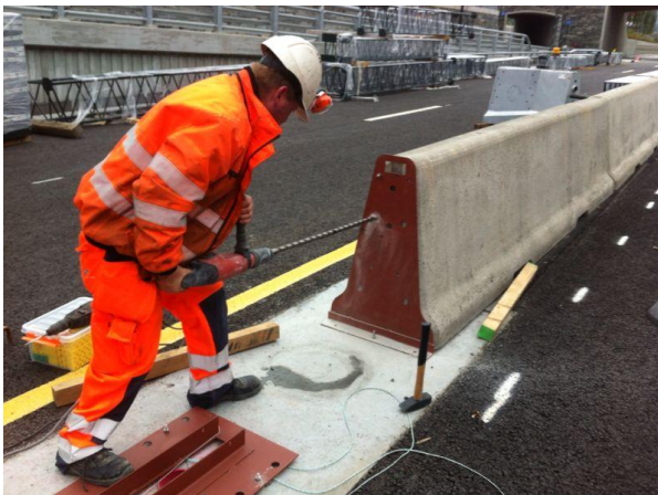
Anchor drilling for transition part
