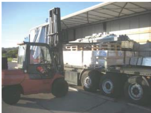
4.1 Abladen des LKW's Unloading the truck
