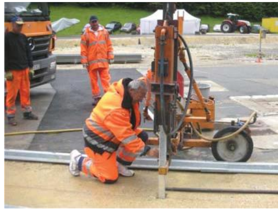
4.8 Rammen der Pfosten Pile driving of the posts
