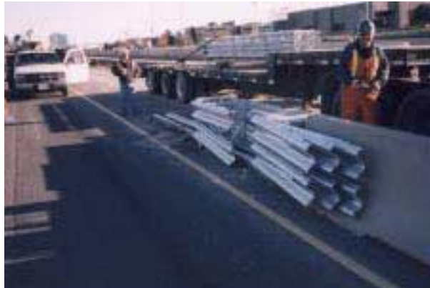
TRACC Replacement in Progress
