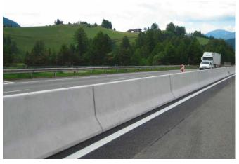
Containment level Working width Impact severity level T3 (covers T2 and T1) W1 (covers W2, W3, W4, W5, W6, W7 and W8) ASI A
