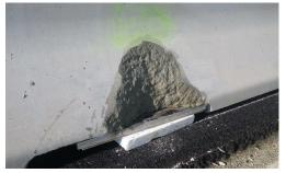
5) If strong cracks (> 2 mm) and/or strong spalling have arisen as a result of the impact and/ or damage / deformation of the coupling is visible, the restraint function can no longer be ensured. In this case the affected elements shall be exchanged for new ones.
