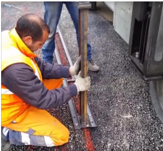
Fig. 9: Driving of the post type IPE 80 with welded plate.
