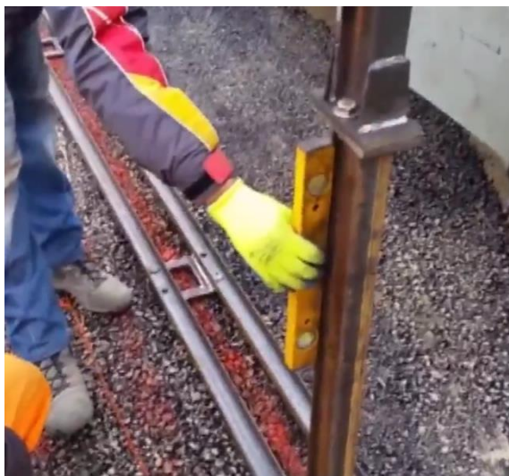
Fig. 11: Check with a spirit level
