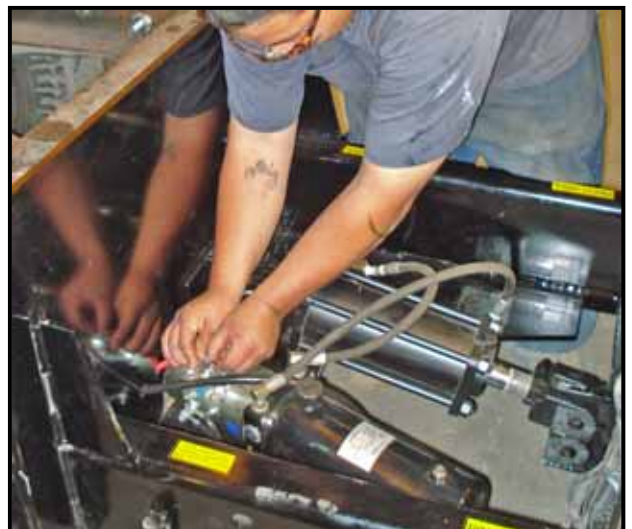
Figure 14. Attached to Support Structure.
