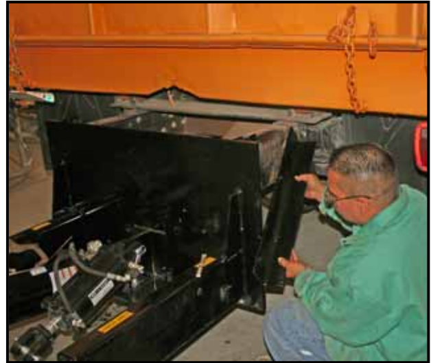
Figure 7. Install side Channel Braces.
