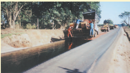
Otta Seals trial, using crushed quartzite with a high amount of fines. The aggregate was applied by a self-propelled chip spreader. (South Africa).
