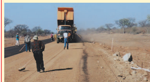
Otta sealing operations. Enough aggregate is essential in order to allow the binder to work its way upwards to coat all the particles. (Botswana).
