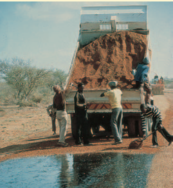
Under the Rural Roads Programme Otta Seals were extensively used, and in combination with labour based work. Natural decomposed granite used as aggregate for Otta Seal was hand screened and applied by hand. (Botswana).
