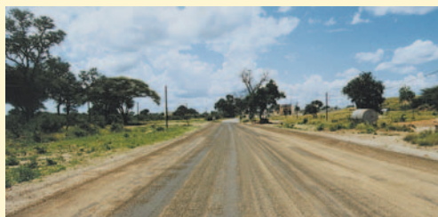
Correct aggregate application rate. (Botswana).
