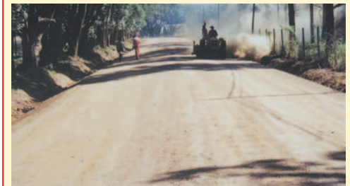
Preparatory work prior to sealing operation, cleaning loose material from the base. (South Africa).
