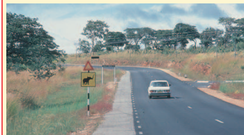
A bituminous surfacing protects the base course layer and provides good riding quality. Hence, low operational costs. (Zimbabwe).
