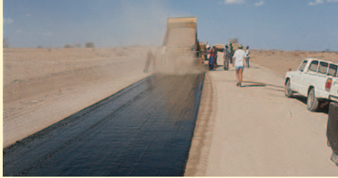
The possible use of natural occurring gravel, including the fines, are some of the factors that favour the use of Otta Seals. (Kenya).
