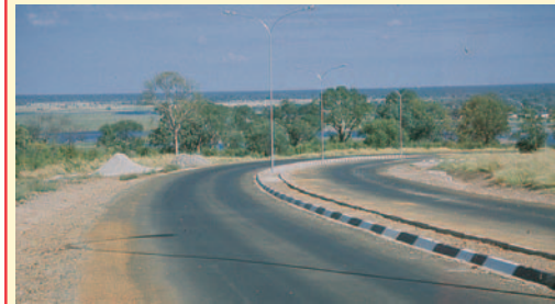
The final product, after 8 months in service of a Single Otta Seal (crushed aggregate) with a sand cover seal on top using fine Kalahari sand. (Botswana).
