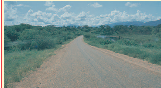
Turkana road, about 20 km north of Marich Pass. Screened quartzitic gravel were used as aggregate for the Otta Seal. After a number of years in service the performance was good. (Kenya).
