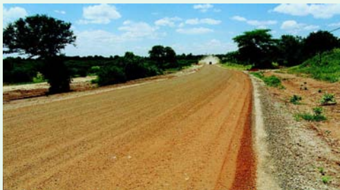
An Otta Seal surfacing 2-3 days after construction.
