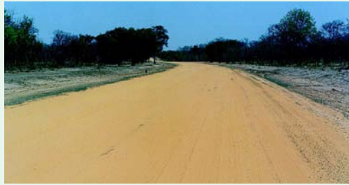
Over application of sand is essential when applying a sand cover seal on top of a single Otta Seal.
