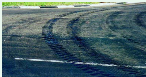
At intersections or roundabouts the occurrence of heavy turning trucks may require adjustments in the Otta Seal design, just as in the case for the more conventional Chip Seal.
