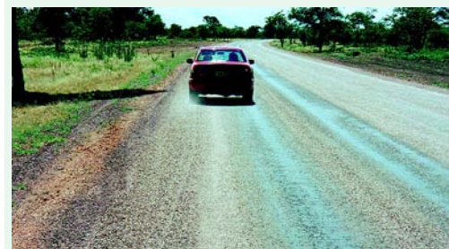
After a period of 8-10 weeks (traffic dependent), the Otta Seal beds down to produce the appearance of an asphaltic concrete premix.
