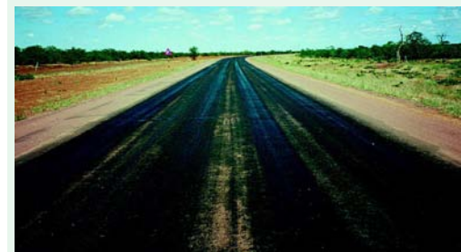
During the first few months after opening to traffic an Otta Seal may exhibit a rich bitumen appearance which initially appears non-uniform and inferior compared to the conventional Chip Seal.
