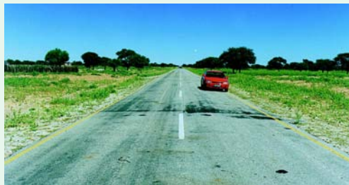
From a cosmetic point of view the transverse joints should be staggered with minimum intervals of 50 metres.
