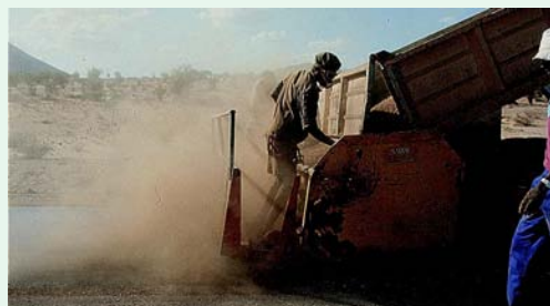
Although the fines content should not exceed 10%, aggregate with fines up to 15% has performed well in Otta Seals.
