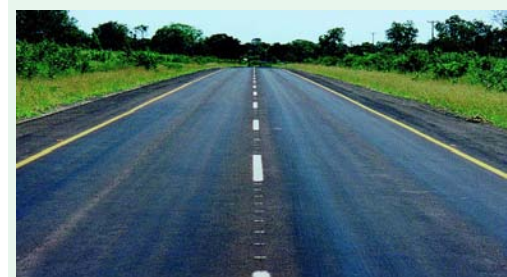
After some months of trafficking, the Otta Seal “beds down” and provides an uniform appearance similar to asphaltic concrete (Kasane – Ngoma road).
