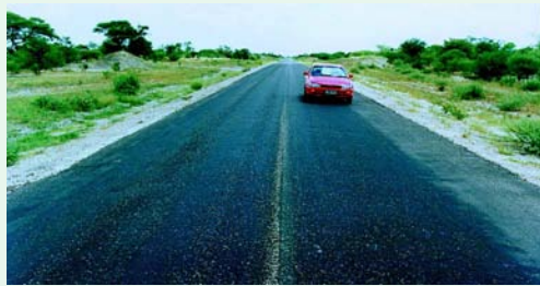
As for any surface treatment, longitudinal joints must have sufficient overlap. Otherwise, this will become the weakest point of the surfacing and will require early maintenance.
