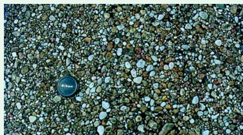
Close-up of the graded aggregate used in the Otta Seal. Note the dense surface matrix.
