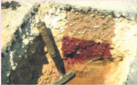
Phenolphthalein reaction in stabilised subbase.
