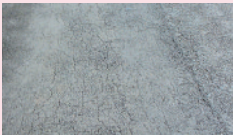
Degree 3 cracking.
