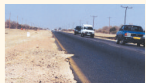
Road with unsealed shoulders.
