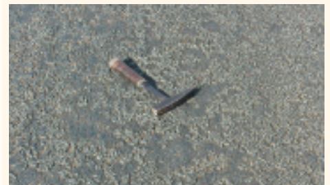
Loss of stone from single seal.
