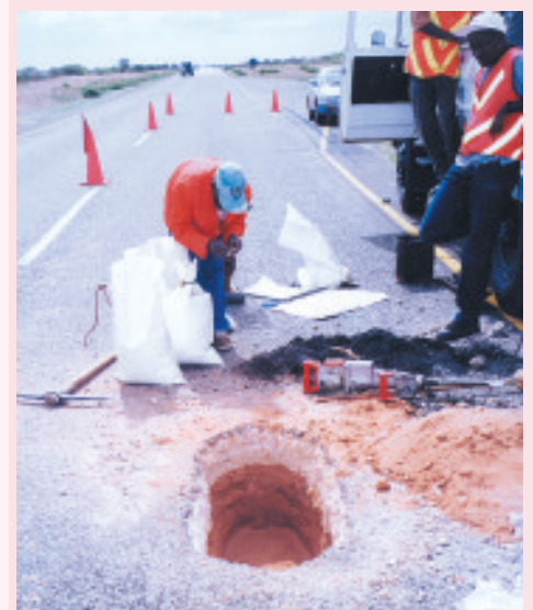
Typical test pit.
