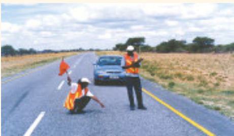
Visual inspection is of vital importance in addressing the pavement condition.
