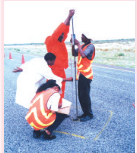
The DCP apparatus, in operation.
