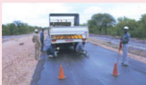
Deflection beam testing.
