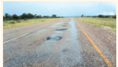
Different degrees of distress in different directions of traffic.
