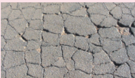
Degree 5 cracking.
