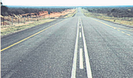
New road - one year after construction.
