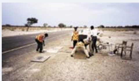
Preparation of mobile weigh bridge site.
