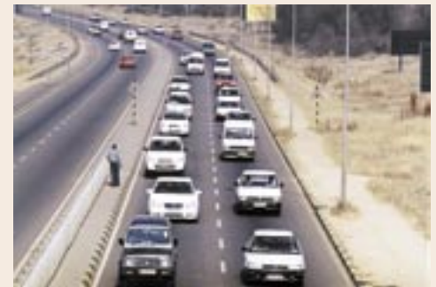
Light vehicles contribute very little to the damage of the pavement.
