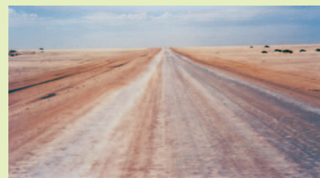
Gravel road on saline ground with addition of salt water sprinkle. Road near Swakopmond, Namibia.
