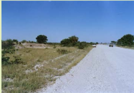
Maron grass, a tough, coarse grass not liked by cattle, found on some road verges can indicate presence of saline ground. Western part of the Kalahari desert.
