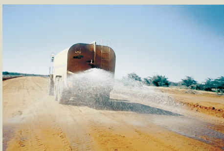
Salt from compaction water is potentially more harmful than salt contained in the materials due to the ability of salt in water to rise more rapidly to the road surface.
