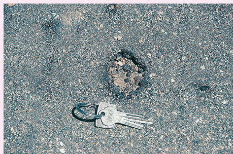
Single salt blister, exposing the base layer.
