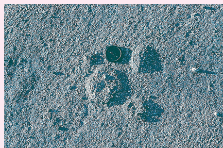
Salt dome, which will break under traffic and
