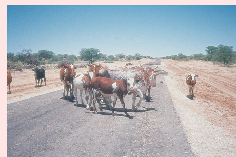
Cattle will congregate and leak salt from the road shoulders if salts are present in materials. This causes a traffic hazard as well as erosion of the road shoulder.
