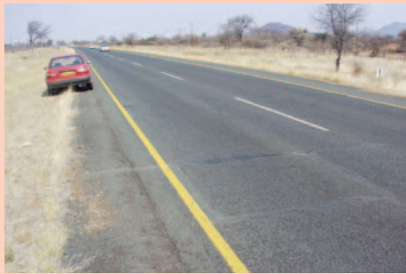
A traffic counting station in a rural area.
