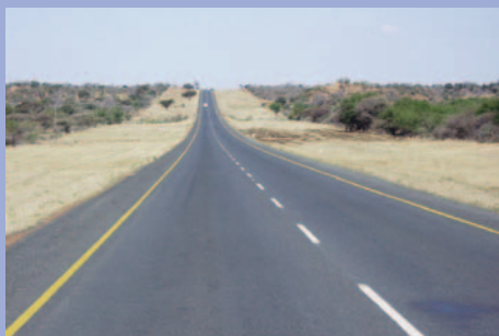
Upgrading of a road is a function of both traffic demand(growth) and prevailing human population to be served.
