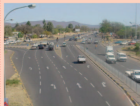
Traffic flow condition influences planning for traffic counts.
