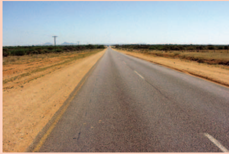
A typical single carriageway rural road.
