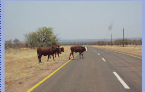
While traffic counting mainly aims at motorised traffic, animal traffic are of importance at design stages for determination of appropriate and safe crossing points.
