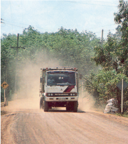
Unpaved roads generate dust in dry weather causing health hazard, damage to crops, vehicles and natural habitats and adversely affecting the safety of pedestrians and vehicles. Is a sealed surface an affordable option? Yes! It certainly can be.
