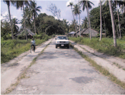
A road where one or more of the seven dimensions of sustainability is missing.
