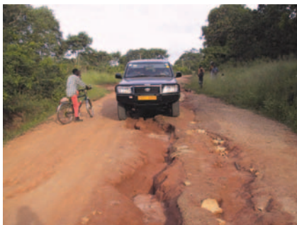
The bulk of the SADC rural road network is still unsurfaced and in relatively poor condition.
