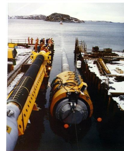
Heidrun Tether Tow & Installation -Holwech et al., FPS 1997 & Engebretsen et al., OTC 2002
