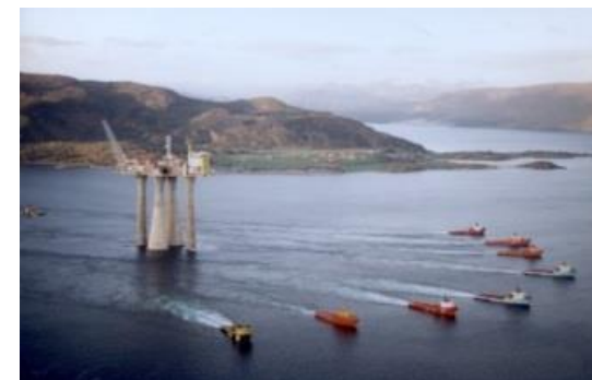
Towing phase for offshore structure
